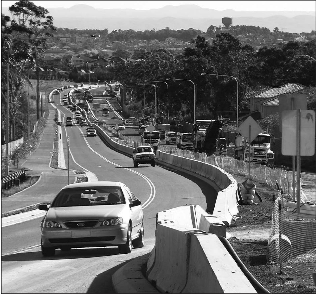
This urban area road was being widened following property acquisition
