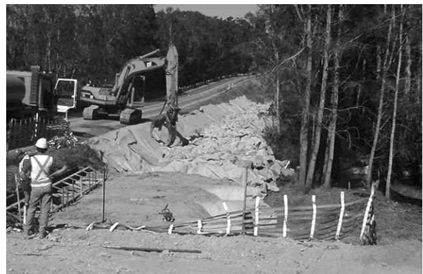
Rockfill keeping Waldron's Swamp clean, Mogo to Moruya widening
